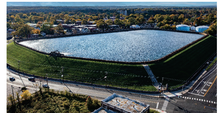
Pennington Avenue Reservoir
