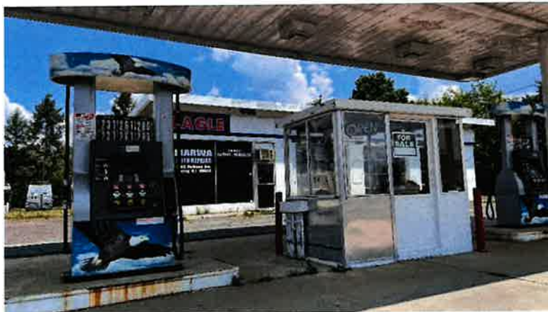
Gas pumps and service booth.
