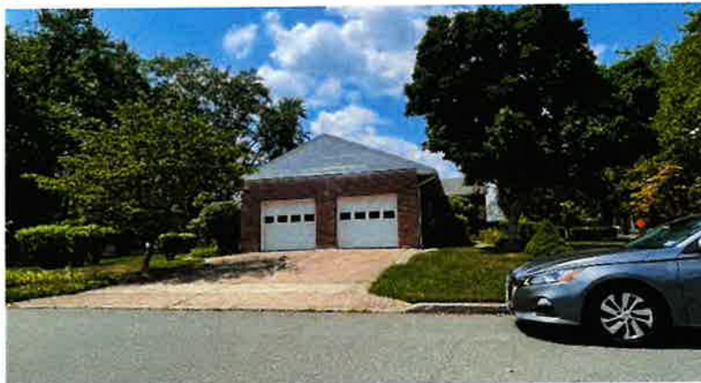
1205 Parkway Avenue from Walter Street.
