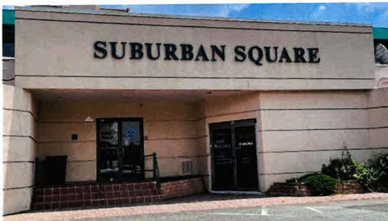
Suburban Square common area and second-floor entrance from rear parking lot.
