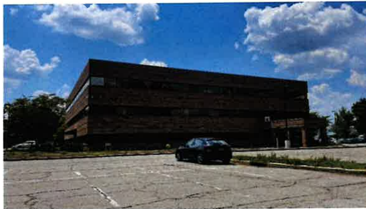
Building rear façade and parking lot.
