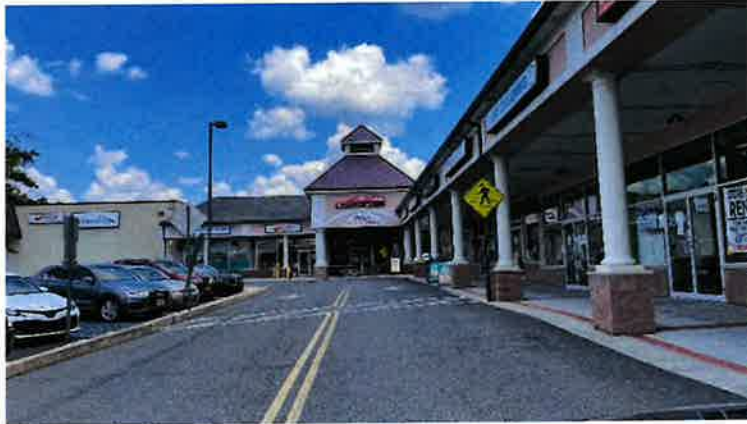
Serenity Plaza from interior driveway.
