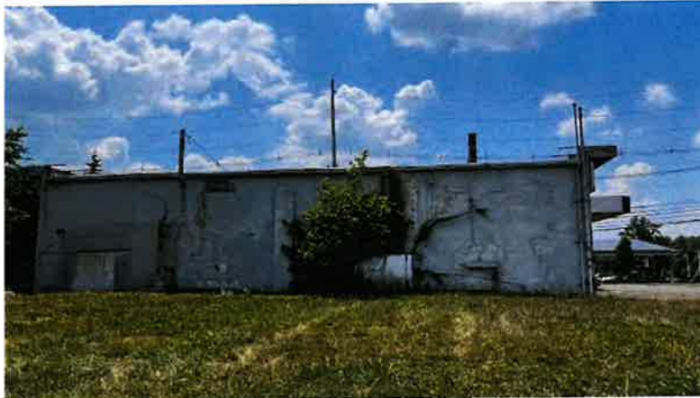
Rear façade from side yard.
