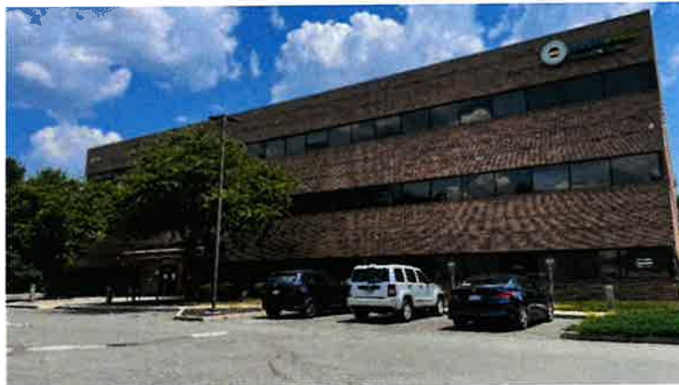
Parkway Avenue frontage.
