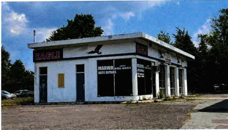
Garage and office building.
