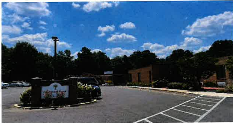
Greenwood House from Walter St
